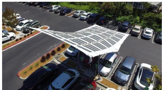
Figure 6- carport with solar flexible panels mounted on top of it [11]
